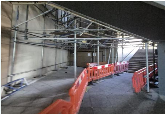
A photo showing Crash Deck Scaffold At 90% and in progress to completion
