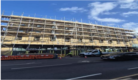
A photo of Front Elevation scaffold at 100% complete
