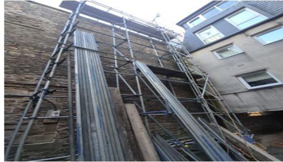
A Photo of Gabel Elevation Hoist Access Scaffolding at 90%
